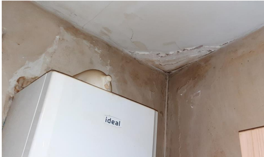
Figure 3 - Leaking ceiling
